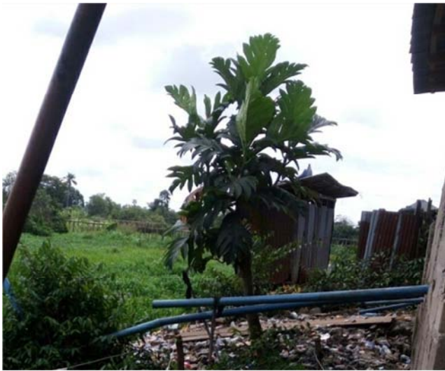
Figure 7. Typical sewage pipes connected directly to the creek.
